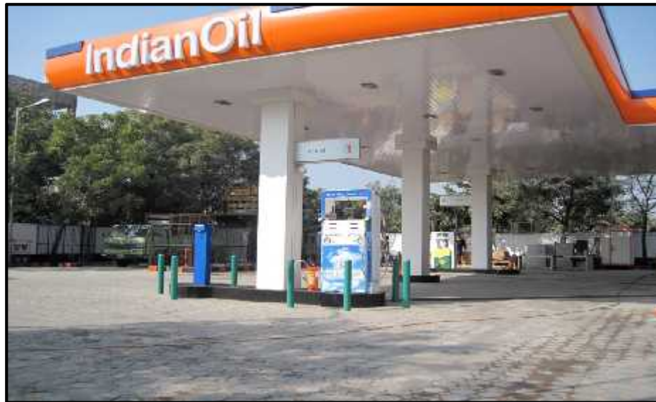
Fig 7.4: Hydrogen/HCNG Dispensing Station at Dwarka, New Delhi
