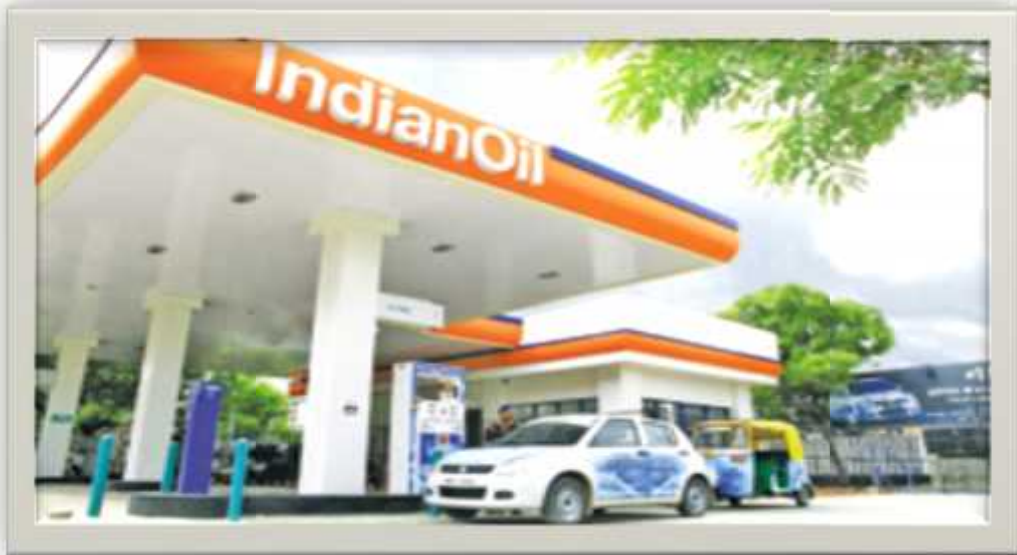
Hydrogen/HCNG Dispensing Station
