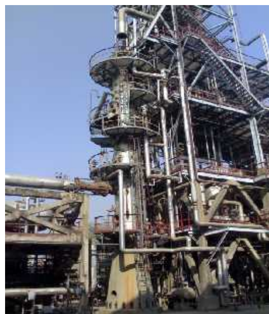
Fig 7.6: TBR Pilot plant Phase III (1.2 m column)
