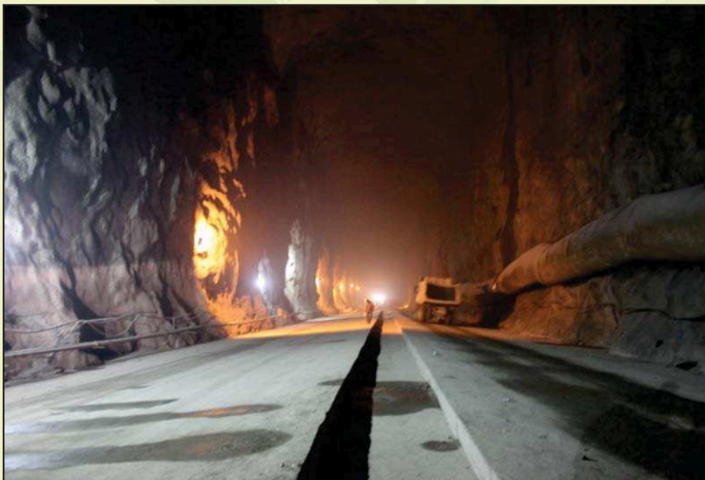
View of one of the four cavern galleries at Mangalore
